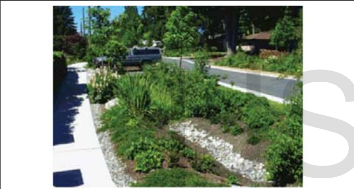
Fig. 3. Example of development of a residential street in the city of Seattle USA with bioretention area [9].
